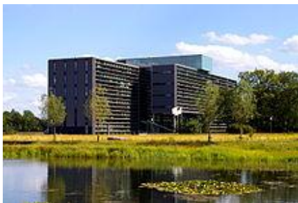
NXP Headquarters in Eindhoven, Netherlands, July 2011
